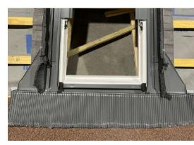
Note: Ensure the correct profile flashing kit is used.
